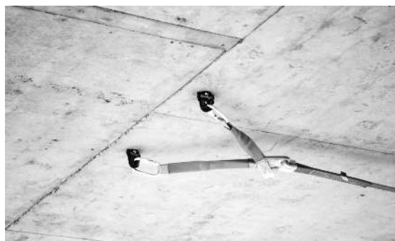
This is how the Lifeline will look when anchored and tensioned at the Webbing Termination end.
