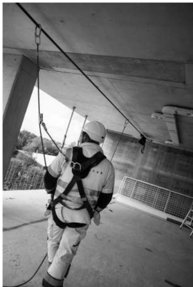
A Temporary Work Restraint System offers long lengths of continuous Anchored travel eliminating the need for clipping.
