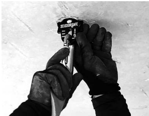
Attach the Anchor to Lifeline Sling to the Anchors with the 25mm Oval Connectors
