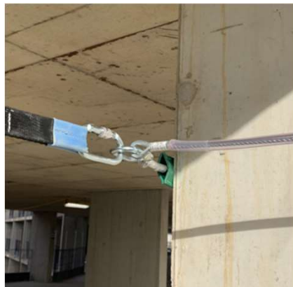
Slings around columns
