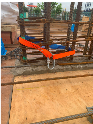
Slings around rebar
