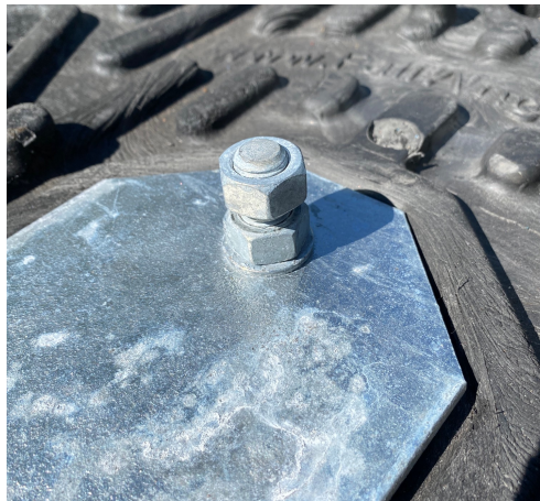
Tighten the first nut then add a locking nut.
