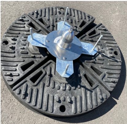
Place the anchor cap on top of the bolts and adjust their position until they line up through the anchor cap holes.
