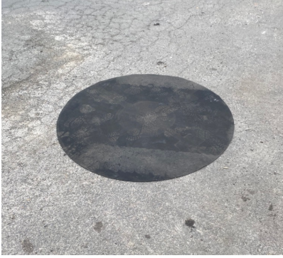
Lay rubber mat on floor, ribbed side down.
