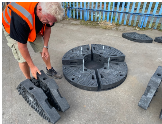
Remove the anchor cap then with the bottom layer of weights in their correct positions, slot the top two layers of weights on top of them.
