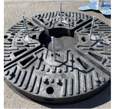
Lay four of the blocks with bolts fed through bottom to form bottom layer
