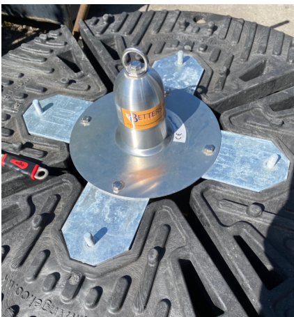
Slide the anchor cap onto the weights , place washer over exposed bolt threads .
